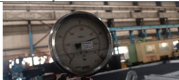
Hydrostatic test control
