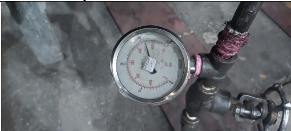
Hydrostatic test control
