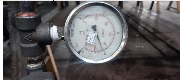
Hydrostatic test control
