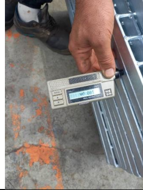
Coating thickness control
