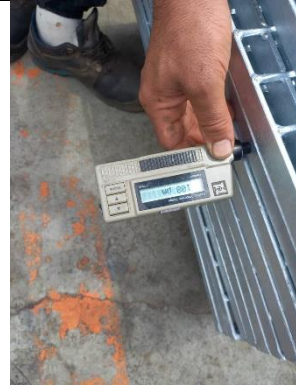
Coating thickness control
