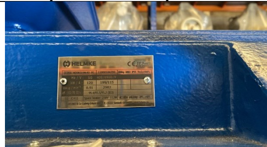
Inspection of 1st Compressor Skid
