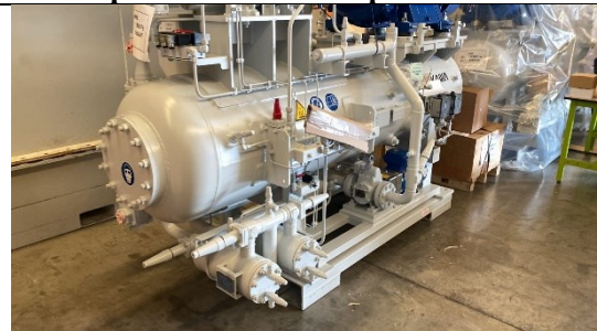
Inspection of 1st Compressor Skid
