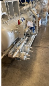
Inspection of 1st Compressor Skid
