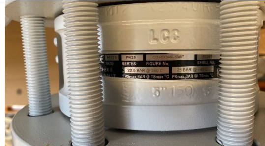
Inspection of 1st Compressor Skid
