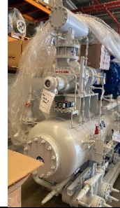
Inspection of 1st Compressor Skid
