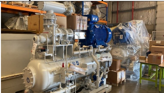
Inspection of 1st Compressor Skid
