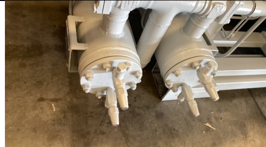
Inspection of 1st Compressor Skid
